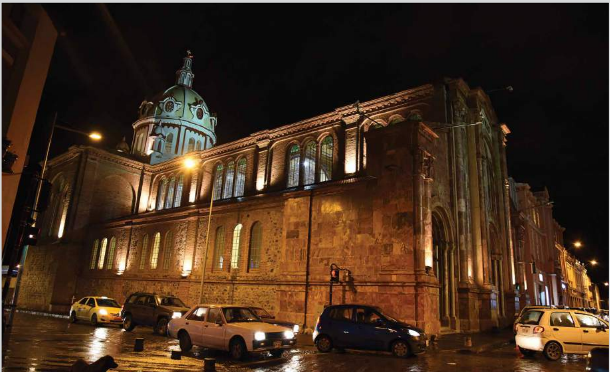
Restoration of San Blas Church
